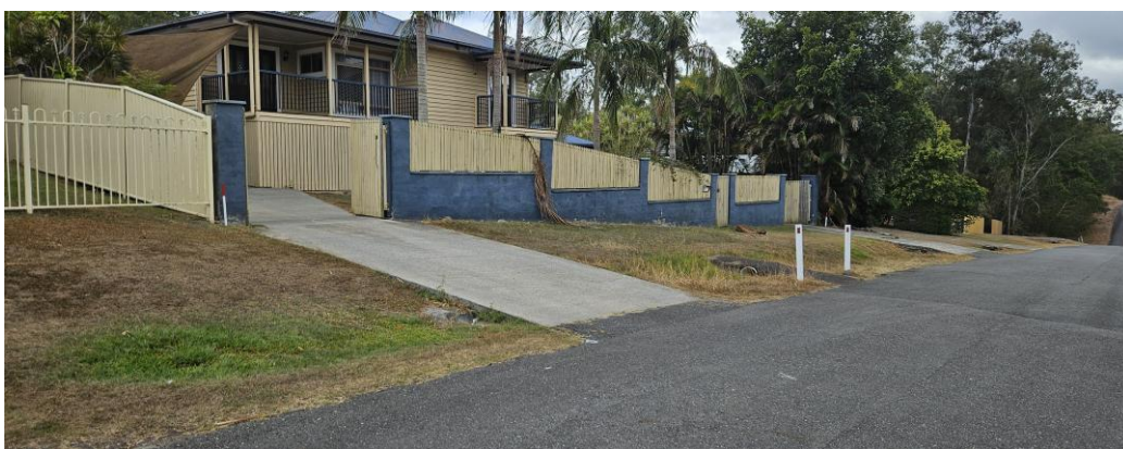
Figure 21 Roadside and driveway interface
